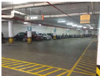
Walkways highlighted at the LG-1 & LG-2 Level for pedestrian safety
